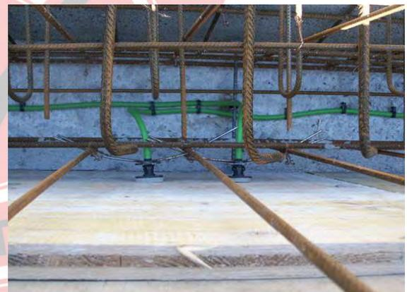
Installing the ventilation hoses inside an **end box**: Important: Ventilation hoses have to be fixed in order to avoid a replacement during the concrete work.
