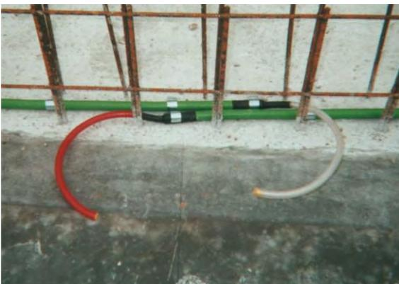
The injection ends shall be placed towards outside the formwork in order to be easily found again. **Two different possibilities are shown:**
